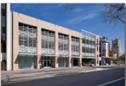
16. Downtown Parking Garage
